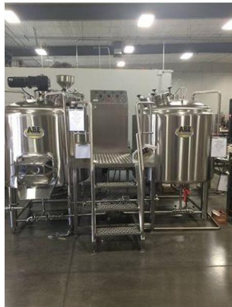
Brewhouse nears completion
