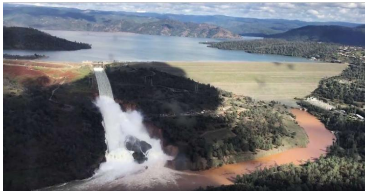
Oroville dam and spillway
