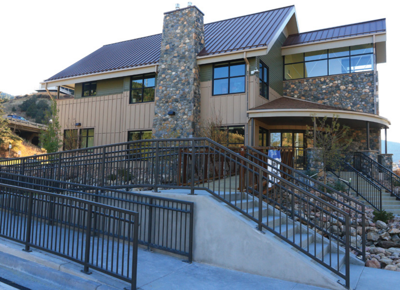
Clear Creek County Health and Wellness Center
