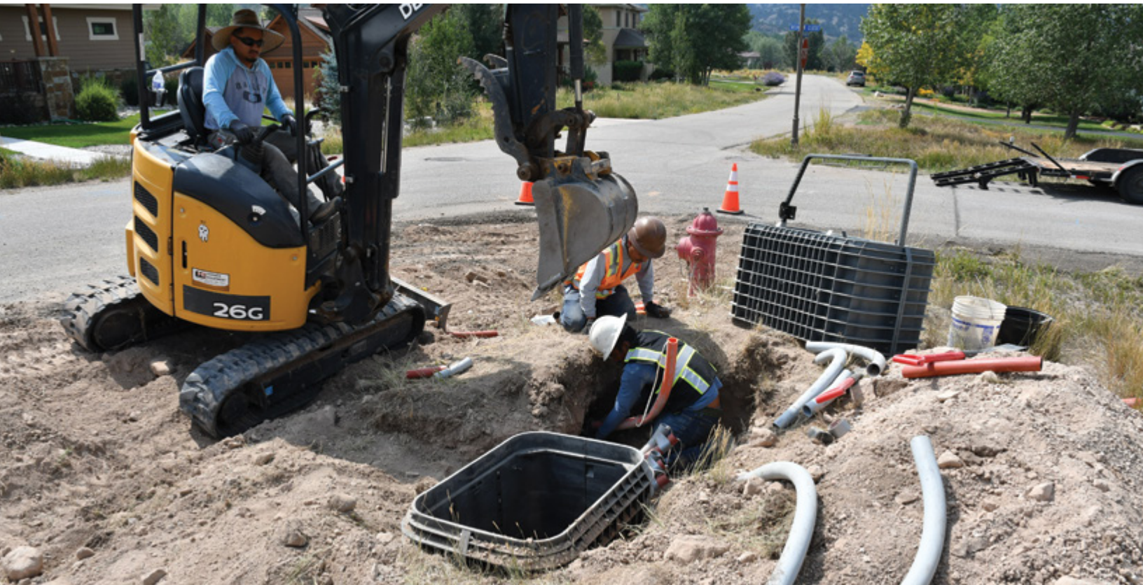
Subcontractor for Comcast installing at Eagle Ranch.
