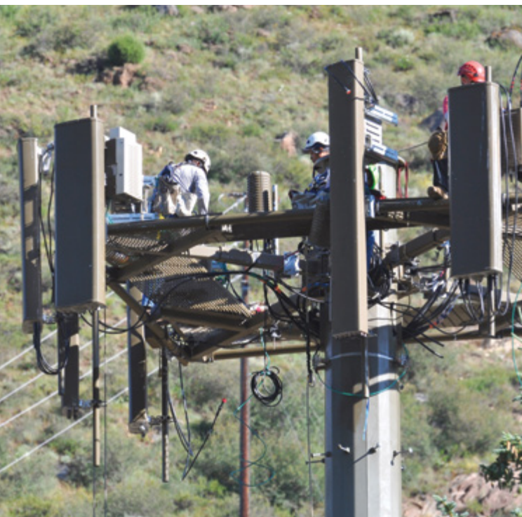
Workers on Cell tower in Vail.
